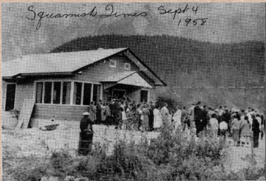
Squamish Times Sept 4 1958 TWO-BED MINIATURE Health Centre, Centennial project for Pemberton and District, opened August 27, has a Public Health office, first aid station, doctor's office, X-ray developing room, Red Cross loan cupboards, two dispensaries, one equipped by doctors from Lillooet and the other by doctors from Squamish, and a large meeting room that will be used by various organizations in the district. There is an automatic oil furnace for heating. Already in use, a young Vancouver dentist, Allan, has been conducting a dental clinic for the past few weeks. He has high praise for the centre's facilities. The building and equipment are valued at $15,000. C.A. 269
